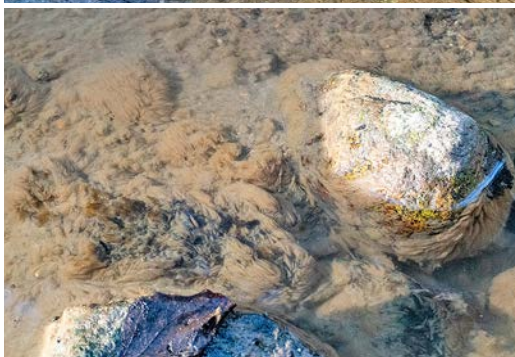
From top to bottom: 1) The clear waters of Stoney Creek upstream of the Rathburn Culvert. 2) Rathburn Culvert (right-hand side) where the heavy growth of algae in the water flowing out of the culvert is visible. The almost vertical grey pipes in front of the culvert connect to the Flowlink unit for continuous water sampling. 3) Close-up view of the growth of algae on creek substrate below the culvert. Photos: Utta Gagel
